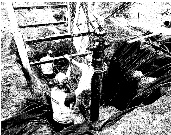
Installing hydrant in front of Rite Aid.
