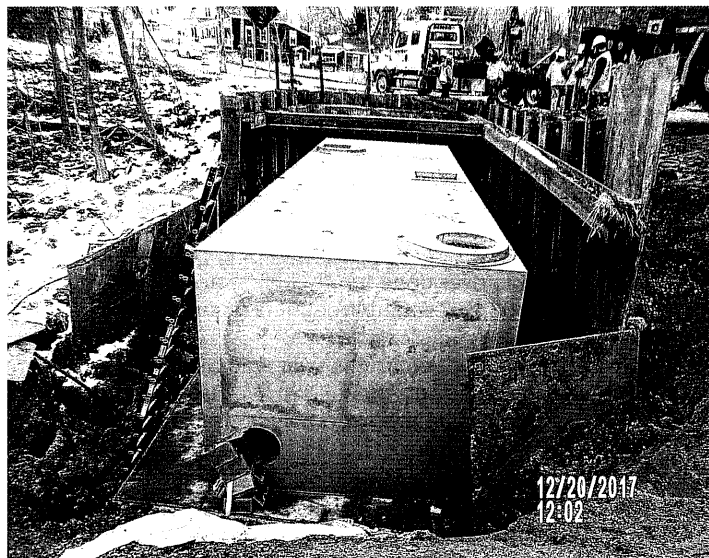
Storm water treatment structure installed on Franklin St.
