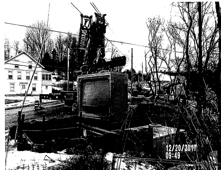
Setting the first section of the day which was the fifth of the structure.
