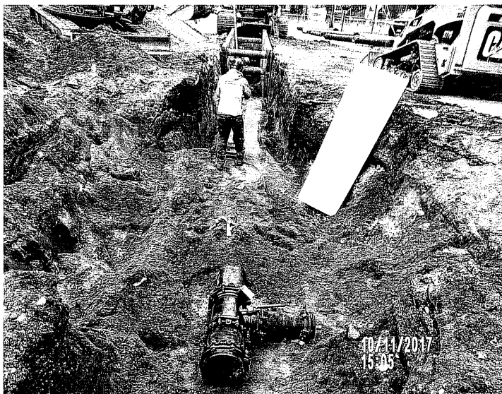
Installed tee for future cross connection on Upper Carver St.
