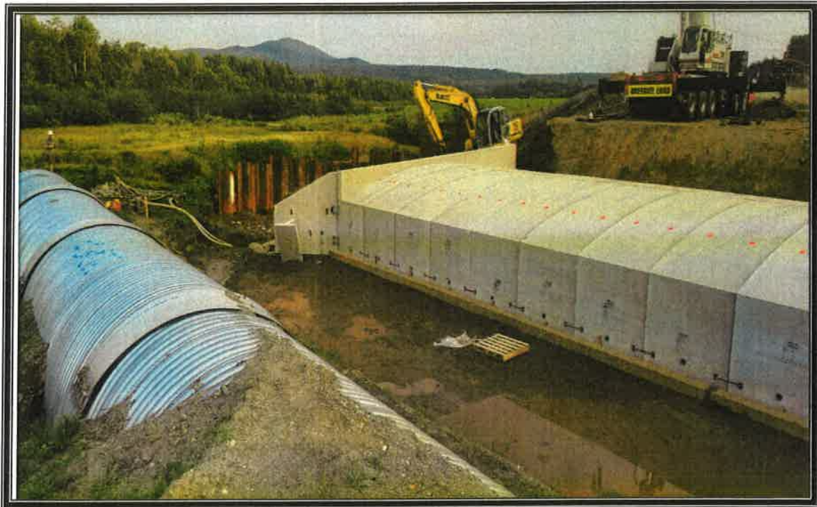
Knowles Flat Culvert Replacement
