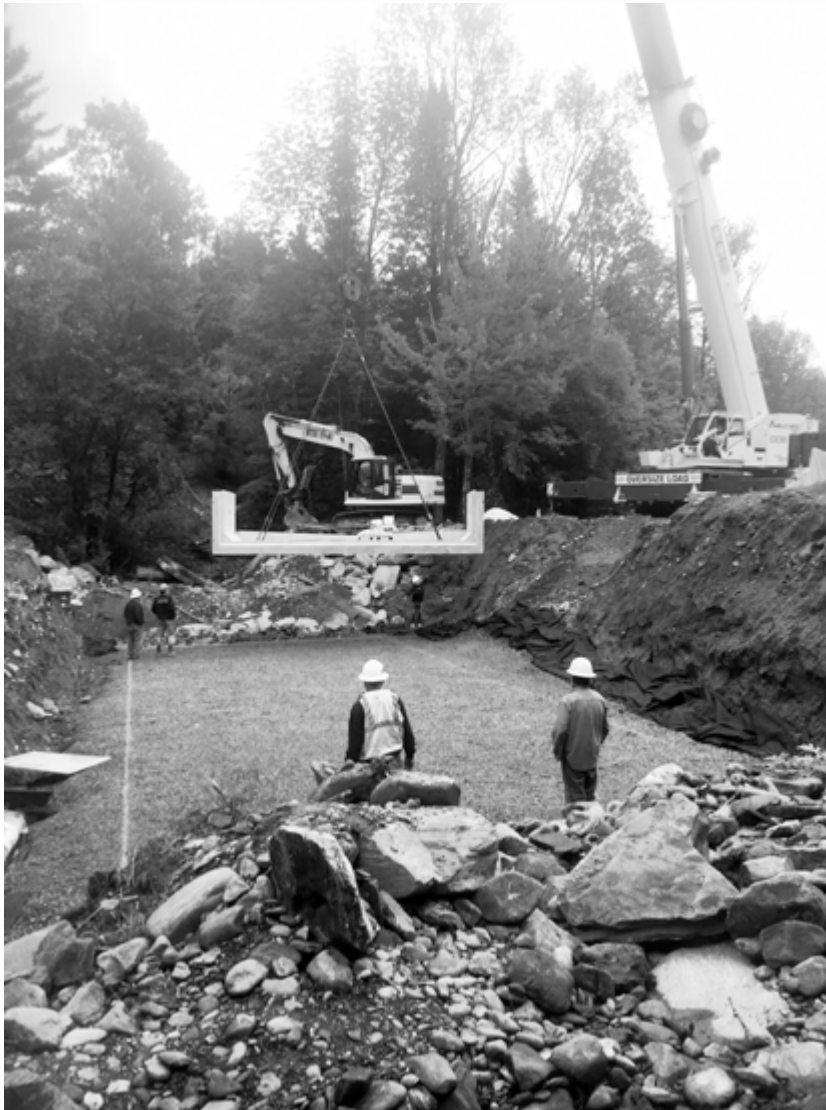
G&N Excavation beginning to install the box culvert on Brook Road
