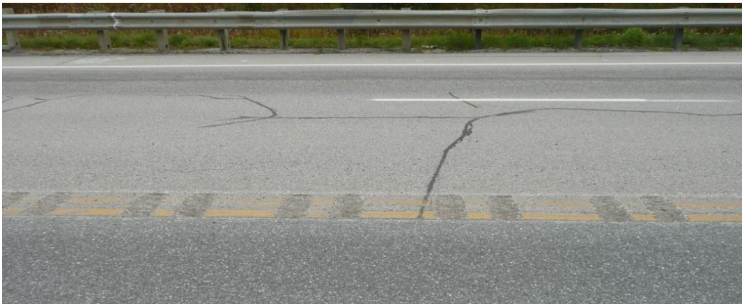
Figure 8: Rumble stripes after milling and sweeping.
