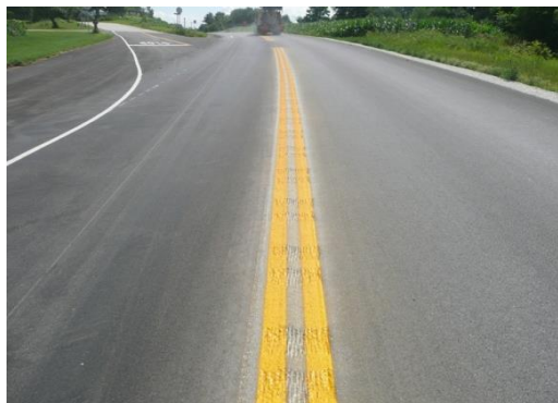
Figure 10: Centerline rumble stripes immediately after painting in Sheldon, VT.
