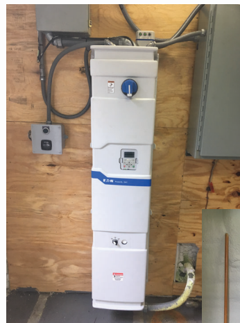
New VFD and Motor at Well #1
