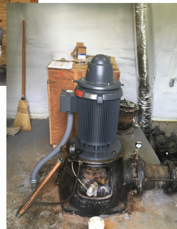
New VFD and Motor at Well #1
