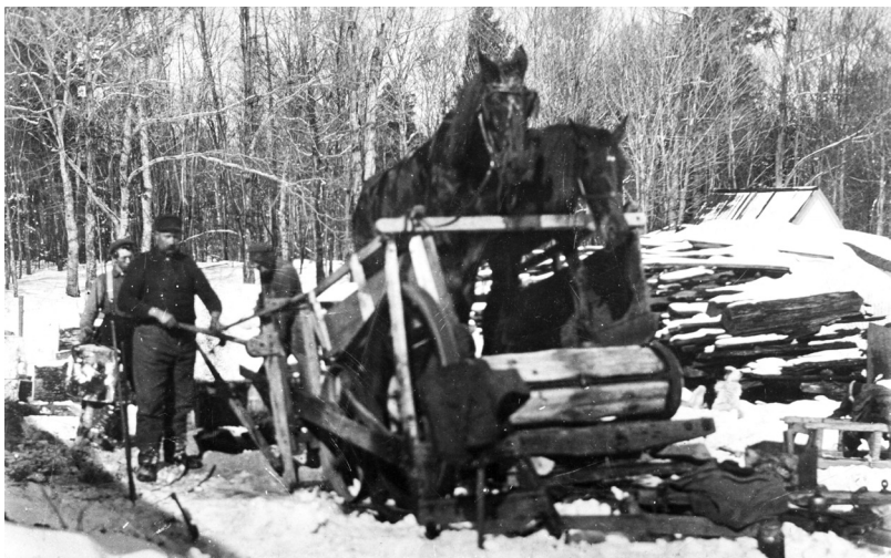
Frank Farnum using his drag saw powered by horses on treadmill at Streeter Farm
