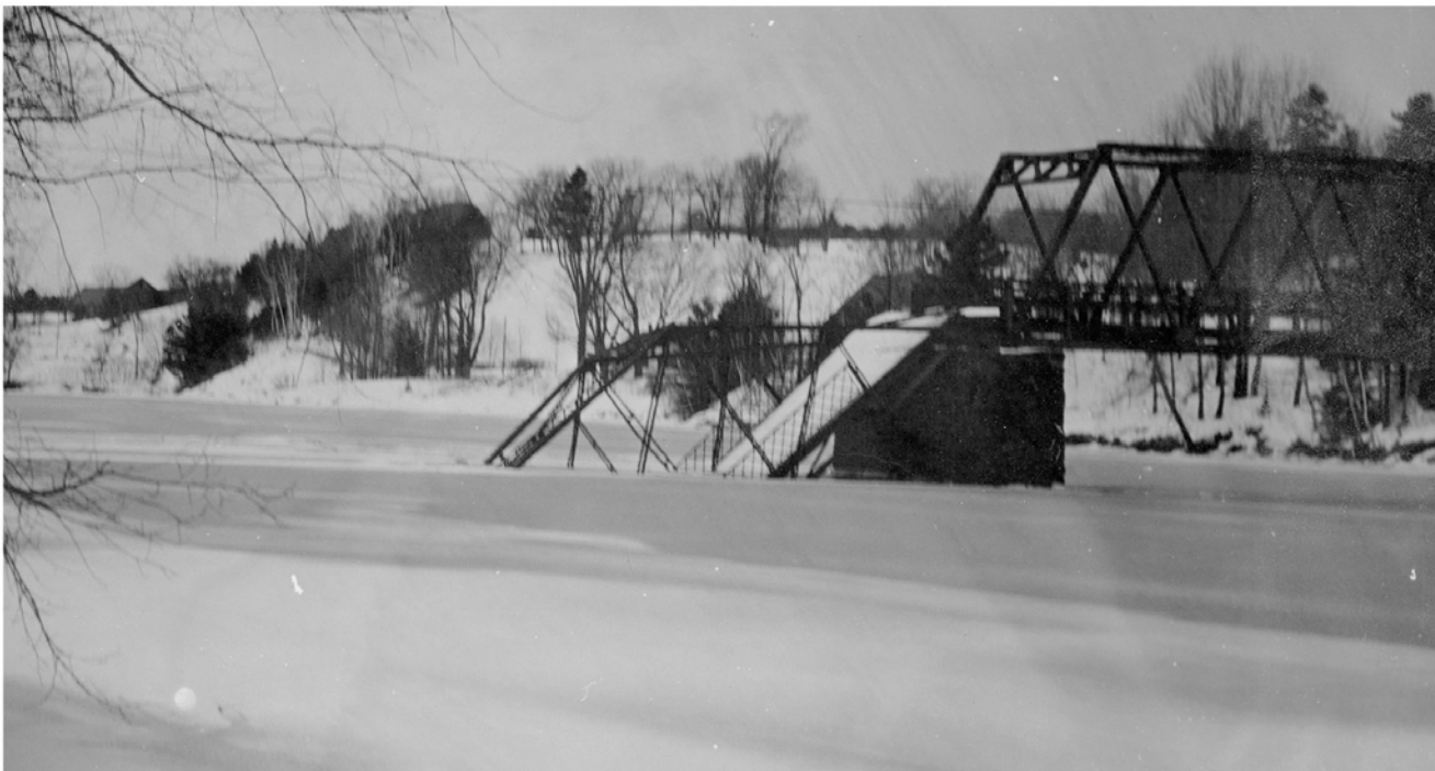
After being damaged in the 1936 flood, the bridge between North Thetford and Lyme was later reduced to foot traffic, and eventually closed altogether. The western span collapsed into the river in 1975. The center abutment is all that remains. (K. Bond Photos)
