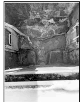
Influent Sewer Structure Clogged with Rags from Items Flushed Daily that Should go in Garbage Can
