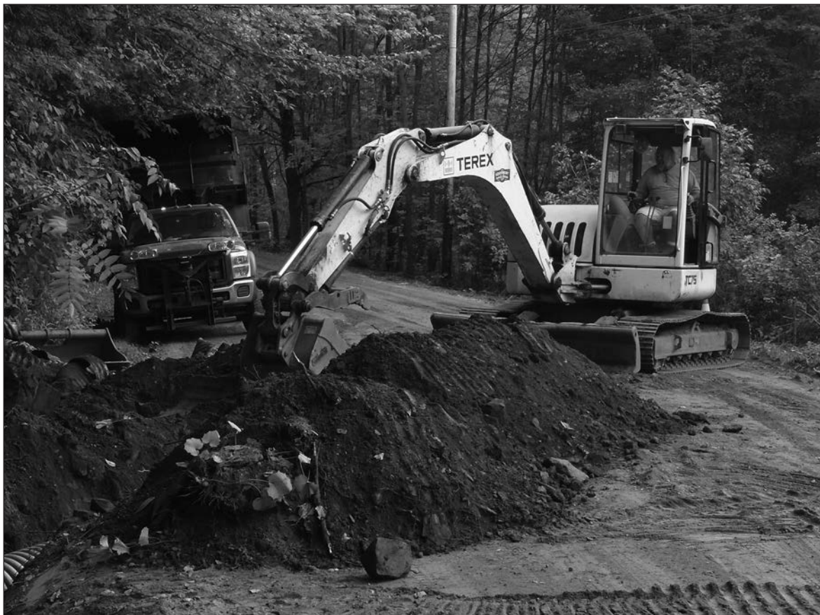
Road foreman Greg Parkhurst replacing a culvert on Foster Hill Road. Photo By Michael Gray
