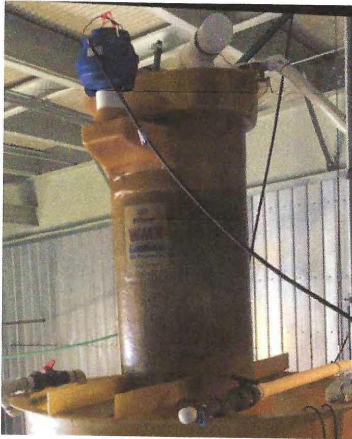
Fig. 5 The gas-stripping tower is mounted on the top of the moving bed bioreactor
