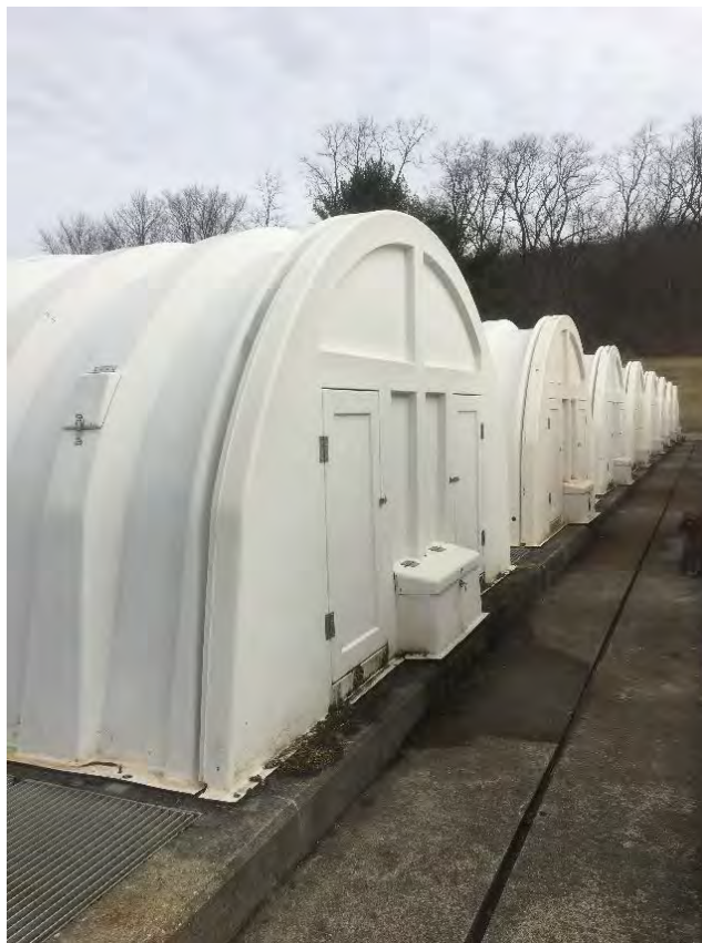
Figure 31. Replacement of rotating biological contactors (RBC) for wastewater treatment, completed by the Town of Bennington with financing from the Clean Water State Revolving Fund (CWSRF)
