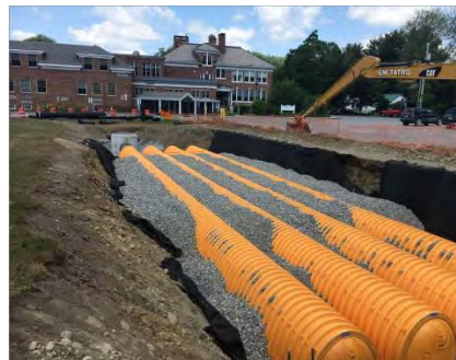
Construction of stormwater treatment practice at Cambridge Elementary , completed by Cambridge Town
