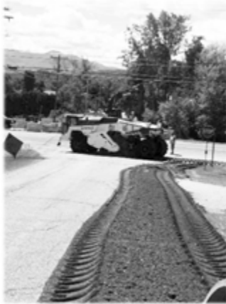
Fitch Hill Road – removing asphalt for new water lines – repaving in 2021
