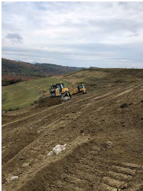
Site Preparation for Plastic Membrane Installation
