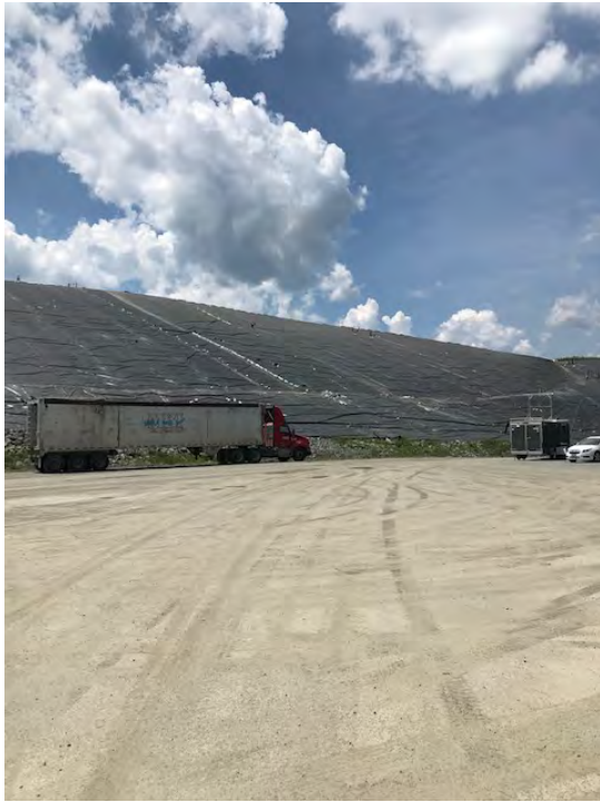
Installation of Plastic Membrane Interim Cap
