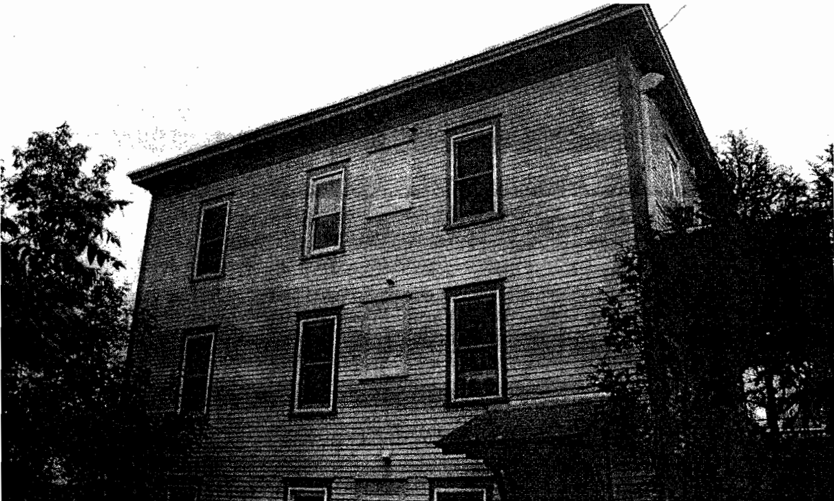
Looking east at back of building. Brackets at eaves and on shed roof entry hood.
