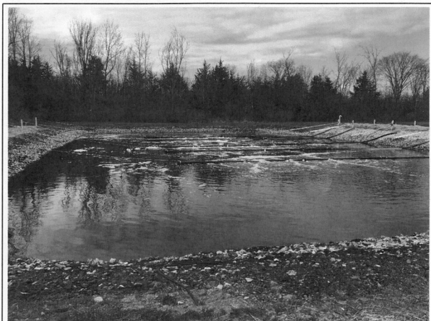
Orwell Treatment Lagoon Aeration System
