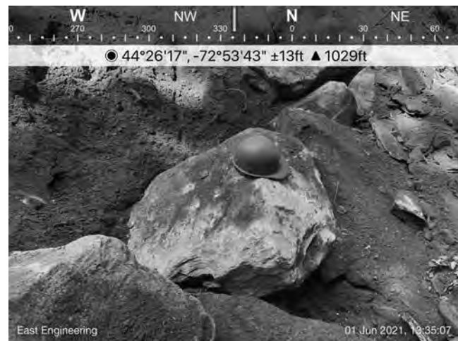
Massive boulders stabilized the FEMA Notch Road slide project.
