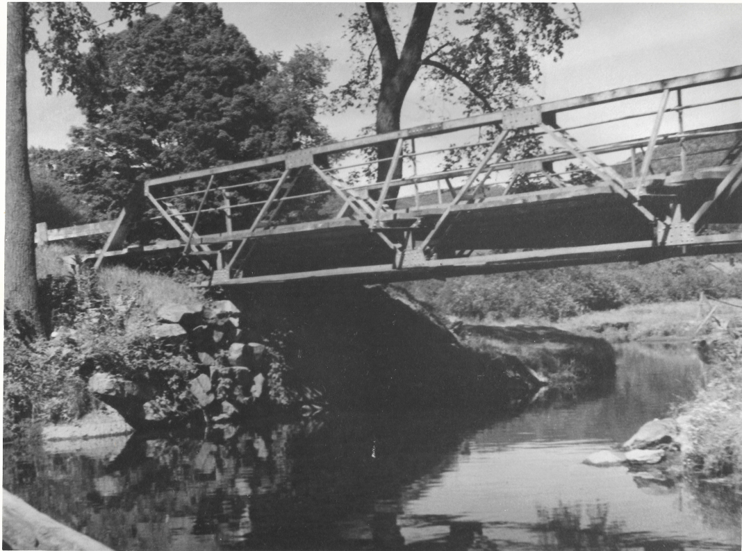
This metal pony truss bridge crossed Lewis Creek on State's Prison Hollow Road (No. 3). The 1941 town report notes $1,043.76 paid to Vermont Steel for the 50-foot span with an 18-foot roadway. It was replaced in 1966 by a concrete bridge, and the old bridge moved to the north end of the Town's Creekside Trail, adjacent to Lewis Creek Farm.
