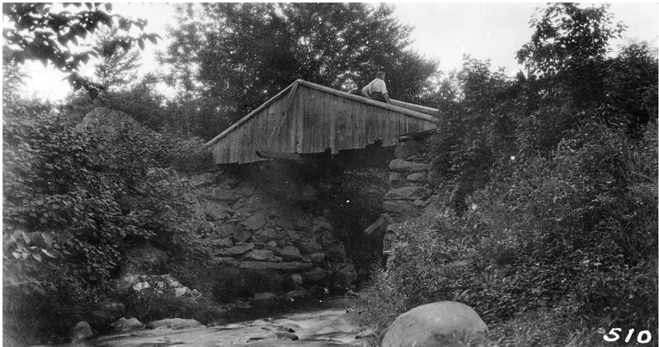
Many town bridges would have been like this timber bridge in town—a simple king's post truss. Board cladding protected the trusses, but also covered up problems. These bridges often washed out in bad storms and eventually were replaced by concrete bridges or culverts. Photo 1922.
