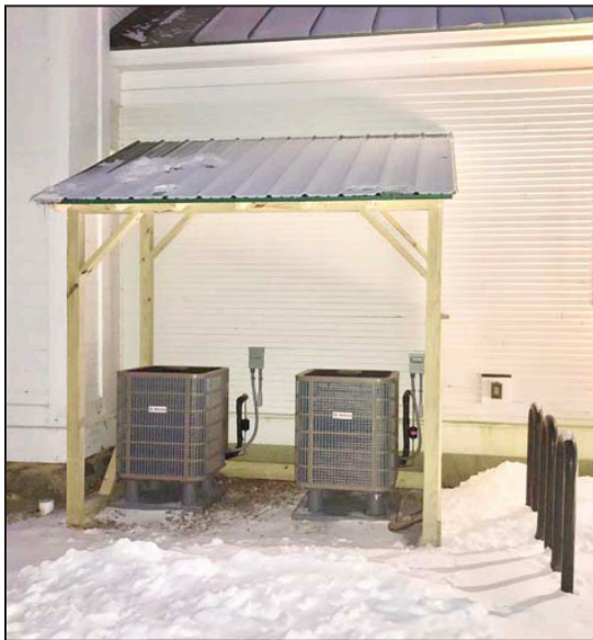
Newly installed condensers for the new heat pump system that replaced the old propane furnances at the Huntington Public Library. Photo: Mary Keller-Butler
