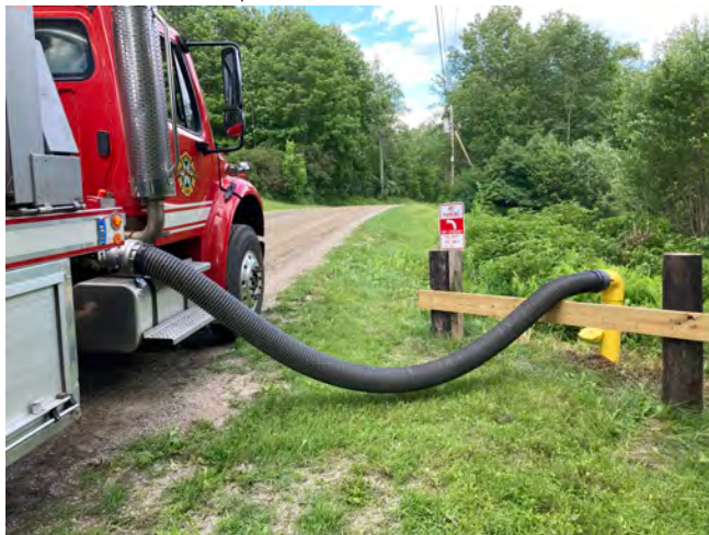
Robbins Cross Rd dry hydrant upgrade
