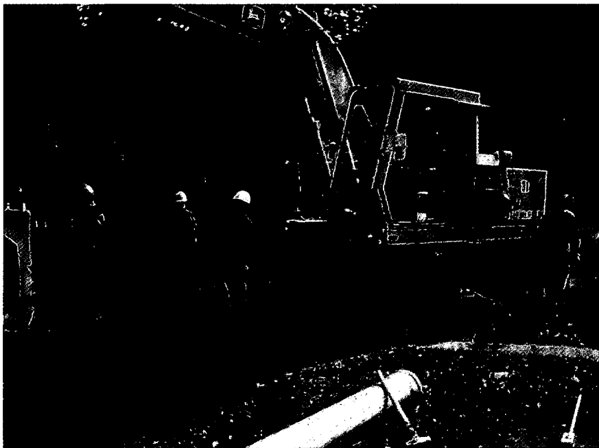
The DPW extended the storm drain and added a new catch basin on Sterling Hill Road.
