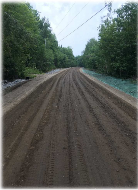
Bornemann Road – new stone lined ditch and hydroseeded shoulder. Better Roads Grant Project 2017
