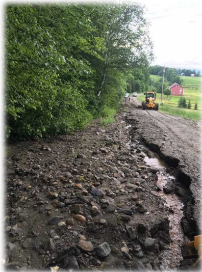
Diggins Road – 3 1/4” of rain in 40 mins; 2 days of work to repair
