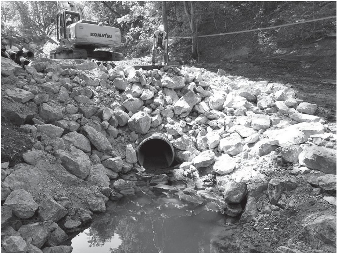
Completion of the Gazo outfall repair project. This is the end of the new outfall pipe
