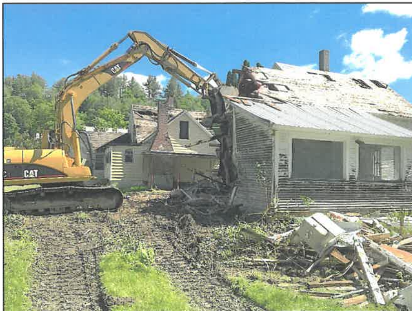
Demolition of 24 East Hill Road property damaged in Tropical Storm Irene and financed in part through FEMA.
