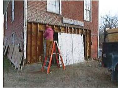
In late November temporary cribbing, new beams and supports, and then plywood sheathing and new clapboards were installed at the southern entrance to stabilize that façade.
