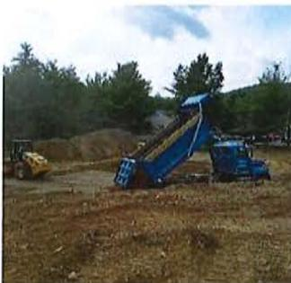
The Highway Department was able to provide all the non-structural and structural fill for the new Public Safety building site. About 9000 yards of fill was hauled from Reservoir Rd. This was achieved in approximately six working days, averaging about 25 loads per truck a day. Supplying this material saved the town a great deal of money in the site work.
