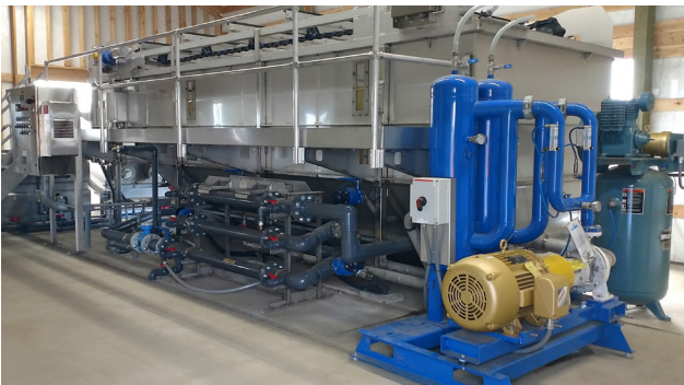
DVO Phosphorus Recovery System Side View.
