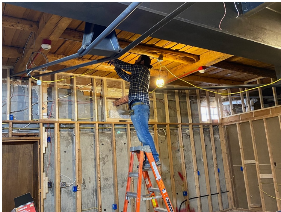
Mike Juris, local electrician installing new electrical and lighting system for town hall basement.
