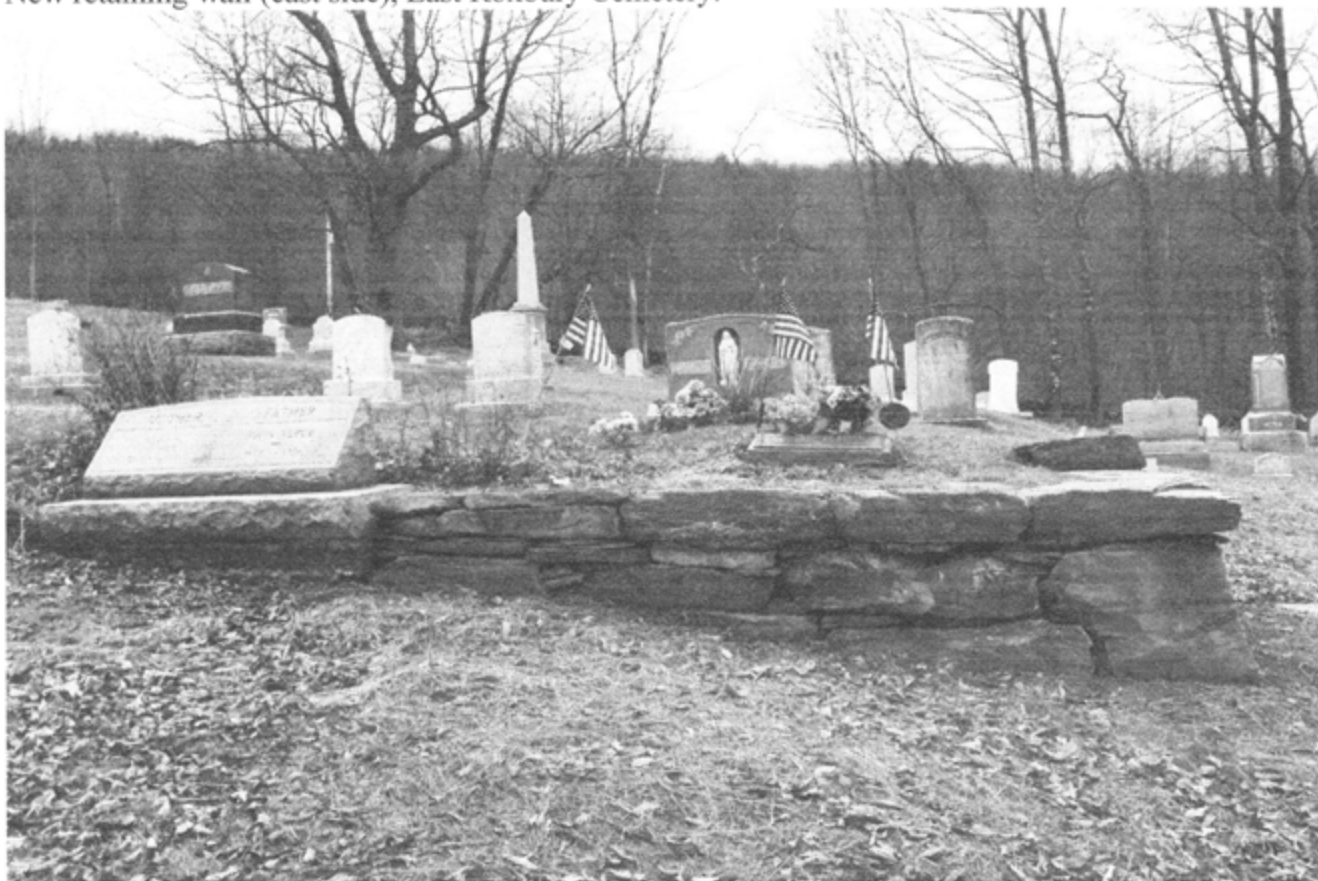
New retaining wall (east side), East Roxbury Cemetery.
