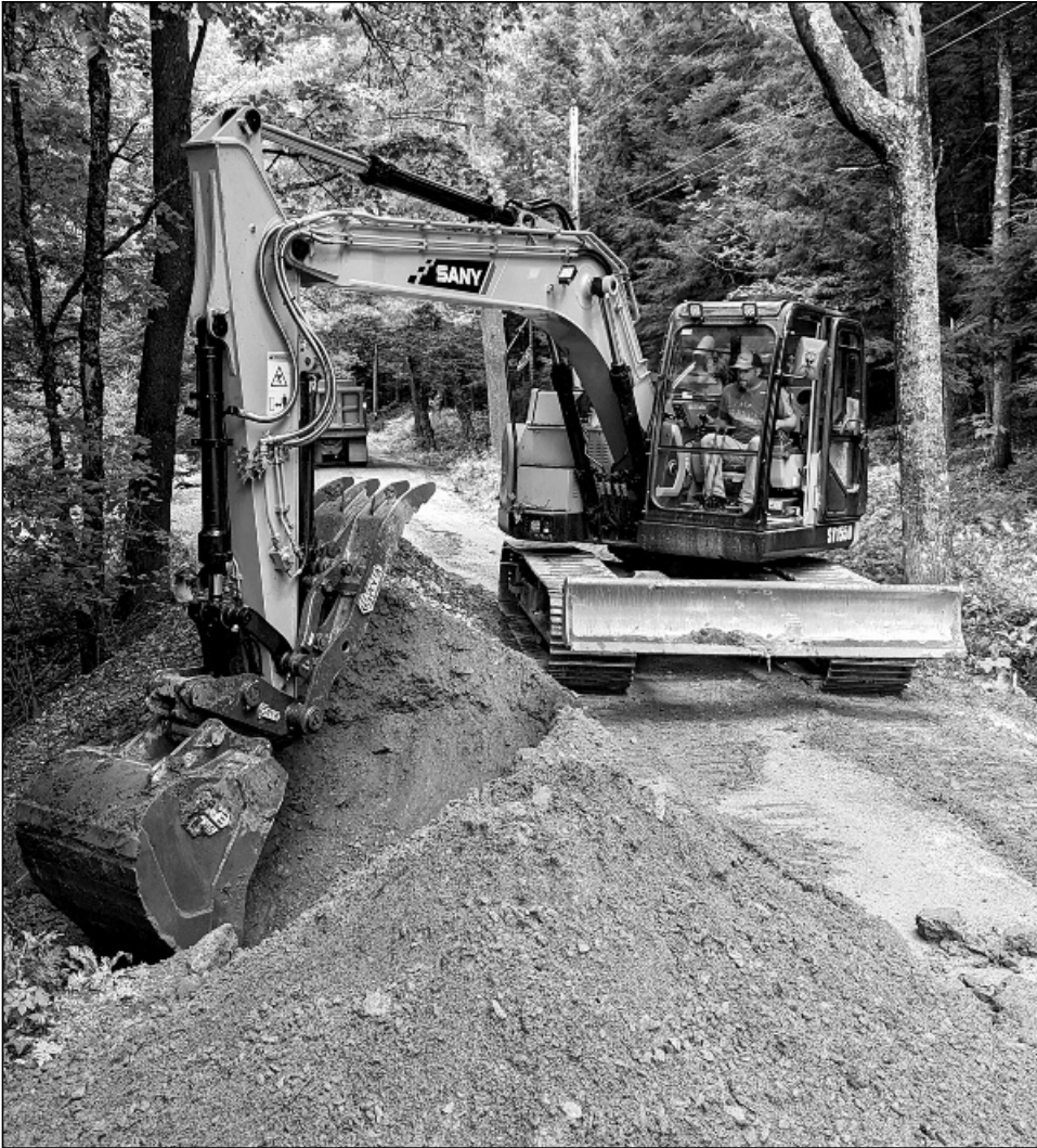
Road Foreman Guthrie Perry replaces another flood-damaged culvert.
