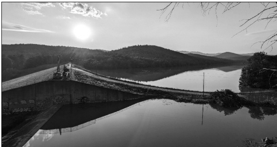
Wrightsville Dam on July 11th: High water crossed the road into the spillway.
