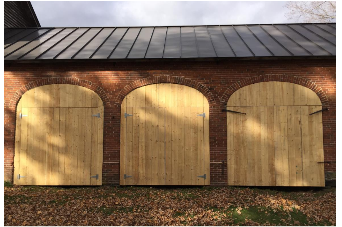
Replicated severely deteriorate doors and hinges
