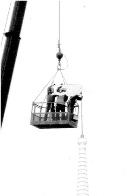
*One of the last tasks in this year's Town House steeple project was re-attaching the weather vane to its mast. Here, Silas Treadway, Adam King, and Joe Cotter place the newly re-gilded, seven-foot, weathervane on the mast.*
