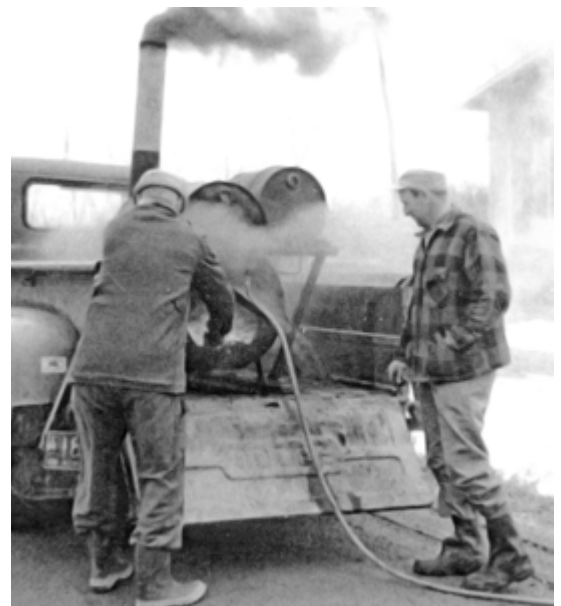
Jasper Santor & Junior stoking a 3-barrel culvert thawing invention.
