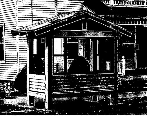
2004, nine new shelters were constructed and one existing shelter was refurbished. All new bus shelters have a durable and attractive timber frame and metal roof and meet ADA accessibility requirements. Additionally, a third size of shelter was designed in the past year. This new version is narrower than the existing shelter designs and will allow CCTA to install shelters in areas previously deemed too small.
