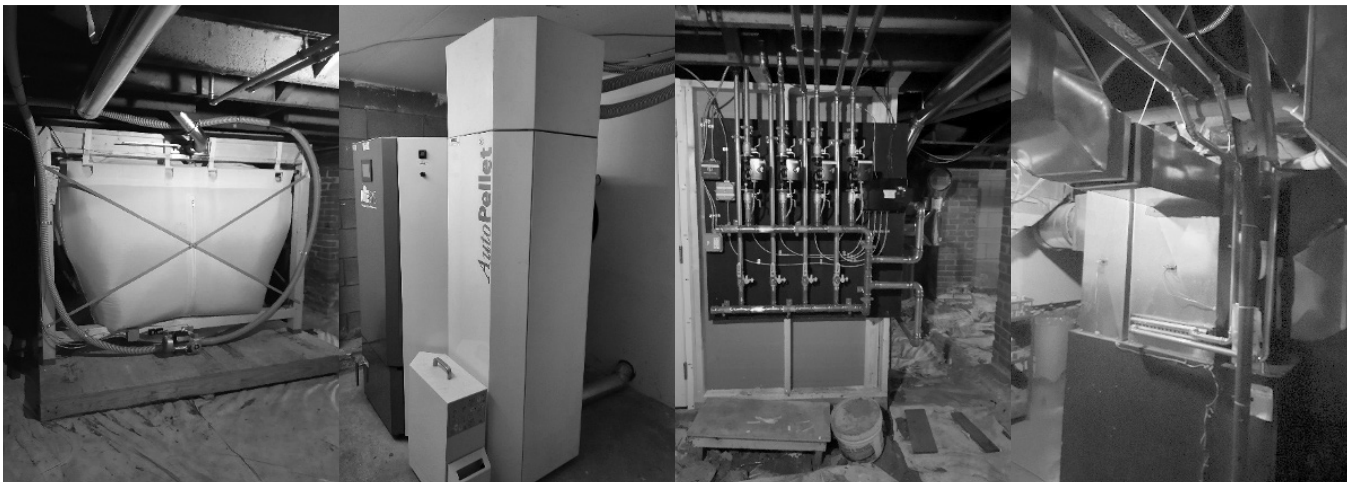
Left to right: Pellet hopper holds 9 tons. Pellet furnace is sleek and automated. Controls on exterior of furnace room. New copper pipes carry hot water to oil furnaces.
