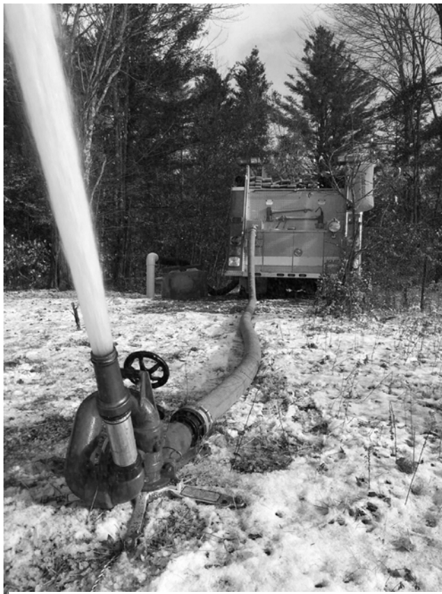
Dry hydrant installation - Fire Brook Rd. Photo credit Chris Pike
